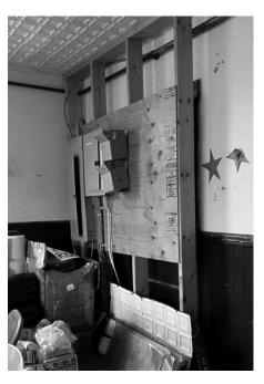
**LEFT:** Green Room ceiling propped after discovery of faulty roof structure. **Center:** Green Room plaster. **RIGHT:** temporary electrical panel installed after flood emergency.
